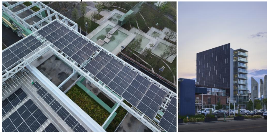
(FIG. 4 Building roof PV system source: Goode Design Network) (FIG. 5 Building PV integration source: Goode Design Network)
