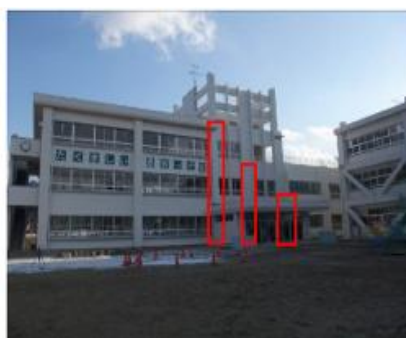
a) Back facade reinforcement
