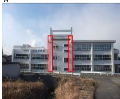
a) Front facade reinforcement
