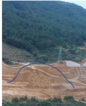
Fig. 1 General view of the slope
