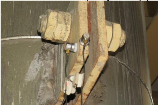
Fig.4 Pipeline vibration test
