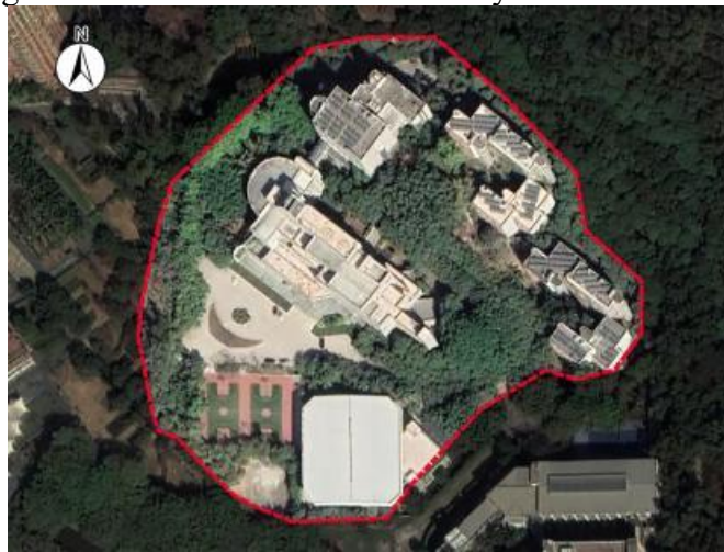
Fig. 3 The current situation of Jinan university Shenzhen campus
