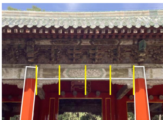
Figure 1. The sparrow brace follows the 1/4 convention.
